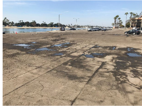
Existing Parking Area
